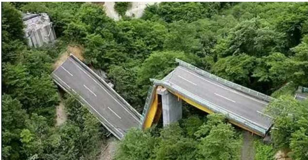
1-rasm. Zilzila ta'sirida ko'prik oraliq qurilmasi shikastlanishi
